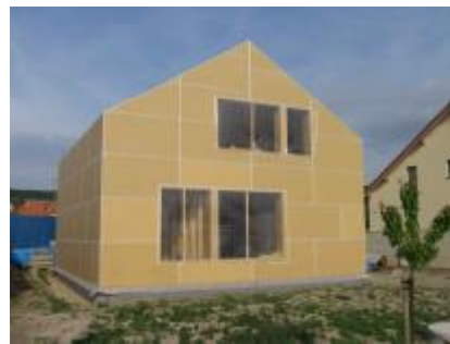
Fig. 8 West view of the Passive House B
