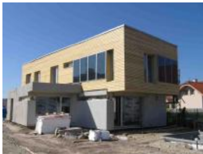
Fig. 3 South view of the Passive House A
